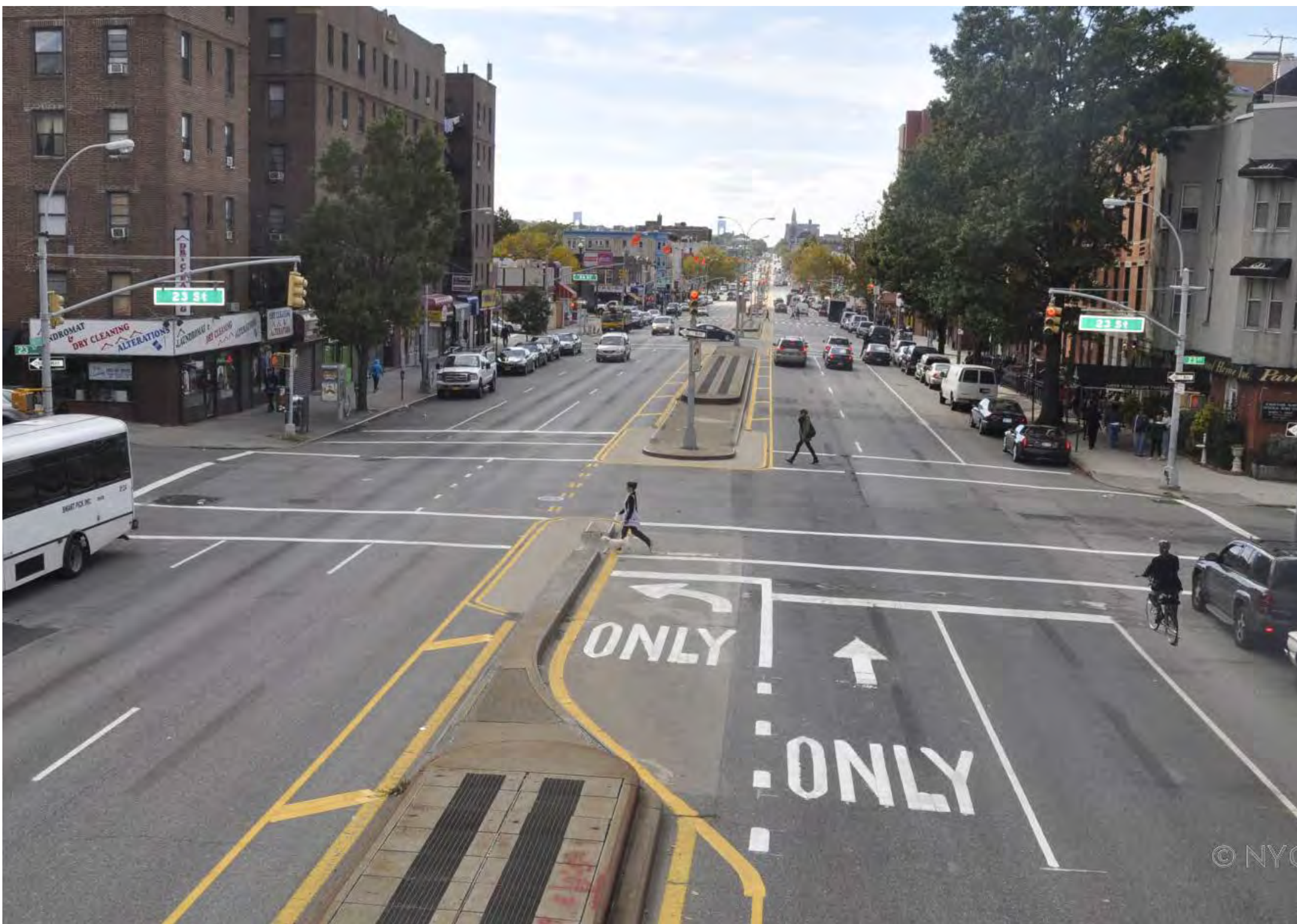
> SMOOTHES TRAFFIC FLOW AT INTERSECTIONS; REDUCES CRASHES AND IMPROVES ROAD CAPACITY (4 TH AVENUE)
