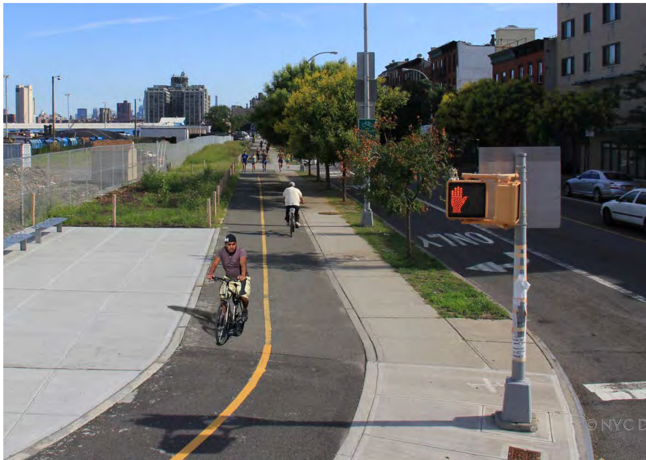
> SEPARATED FROM TRAFFIC WITH PLANTERS, CURBS, OR PARKED CARS (COLUMBIA STREET)
